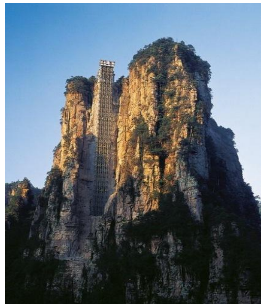
Bailong Sightseeing Elevator
